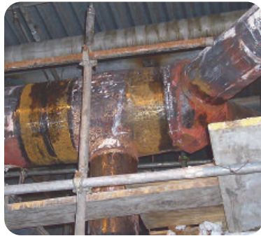
Stress analysis for crotch crack assessment in heavy section wye.
