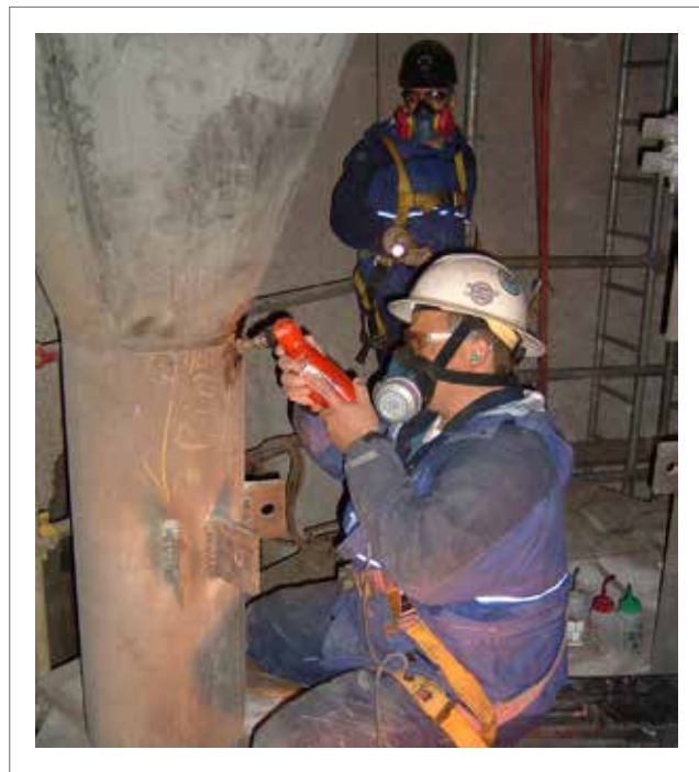
Conducting on-site Field Metallurgical Replication
