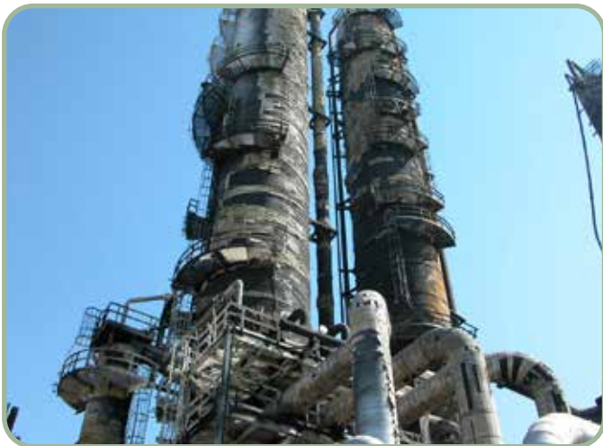
(above, below) Vessel Fire Damage Assessment
