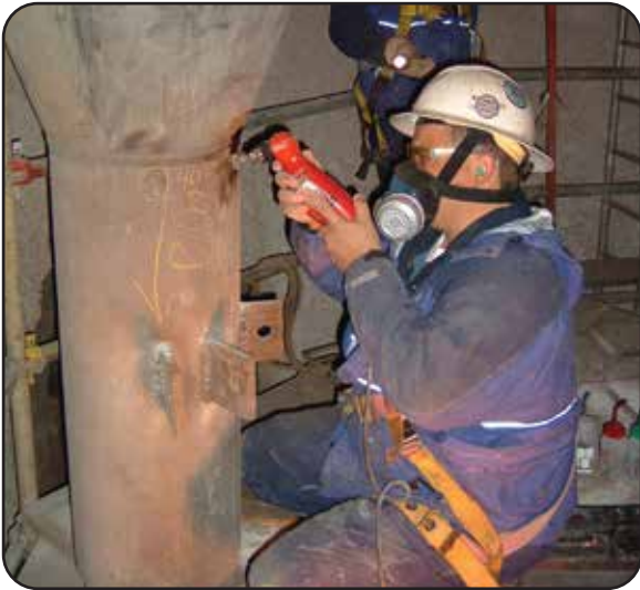
In-situ surface preparation
