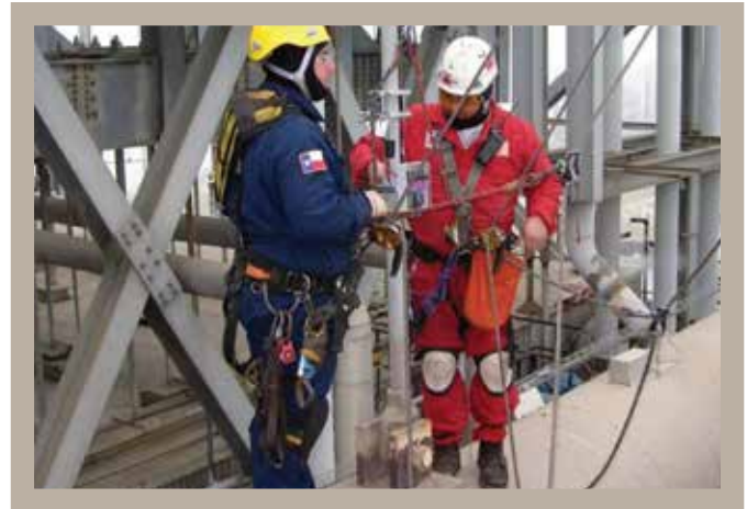
Installation of Pipe Hanger Load Monitor
